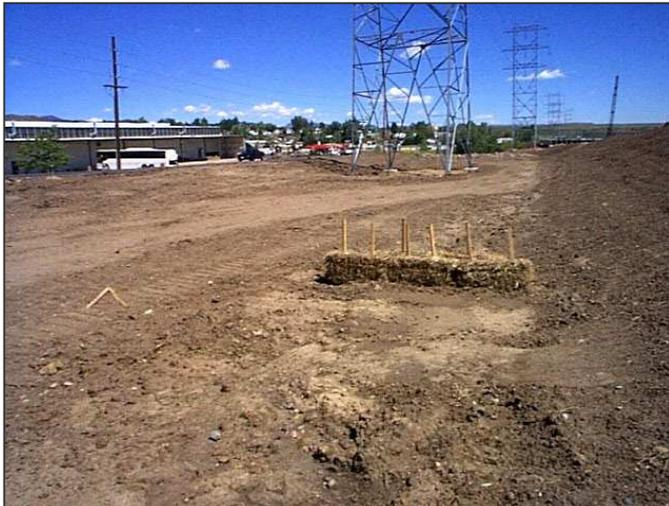
This straw bale barrier was not installed properly because runoff is able to flow around the barrier.
