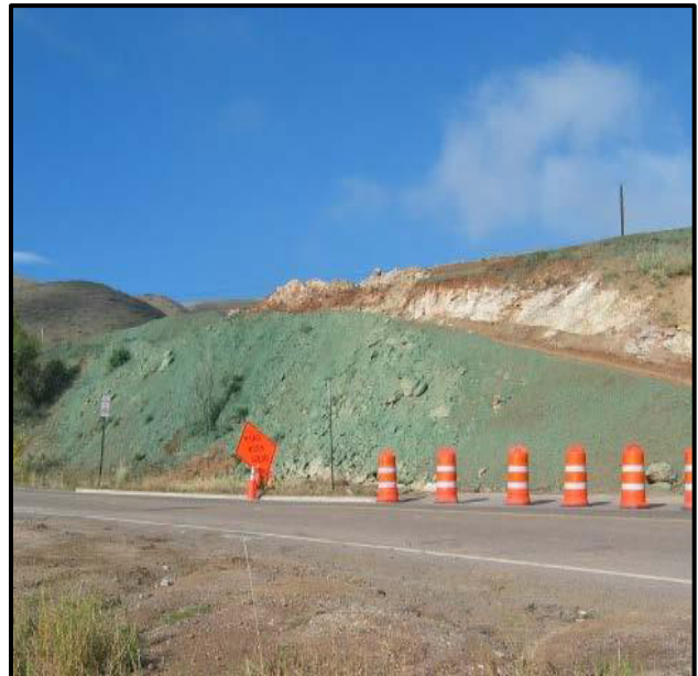
Hydromulch on disturbed side slope
