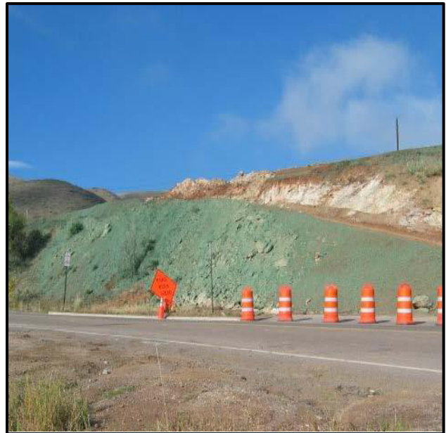
Hydromulch on disturbed side slope
