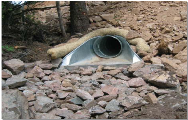
Photograph TOP-1. Riprap outlet protection.
