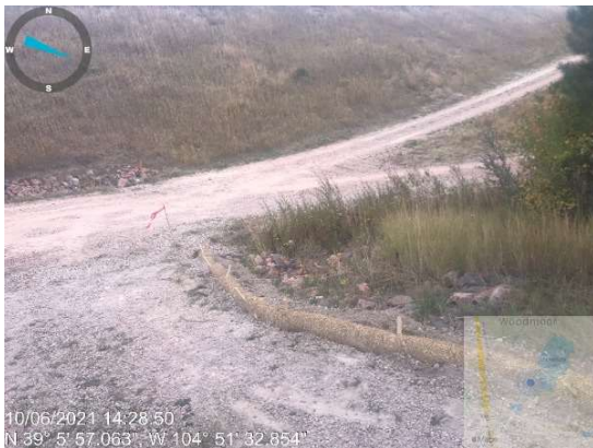
Straw wattle implemented as per plans.
