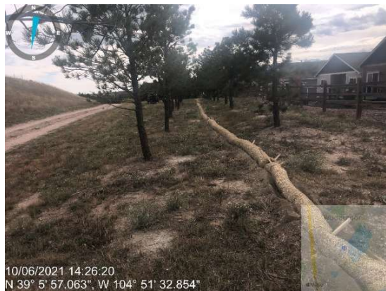
Straw wattle implemented in the rear of lots on Willow Park Drive as per CE1.1.
