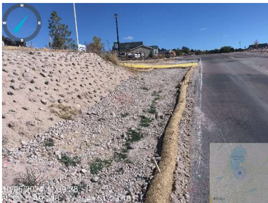
Straw wattle implemented along Lake Woodmoor Drive.
