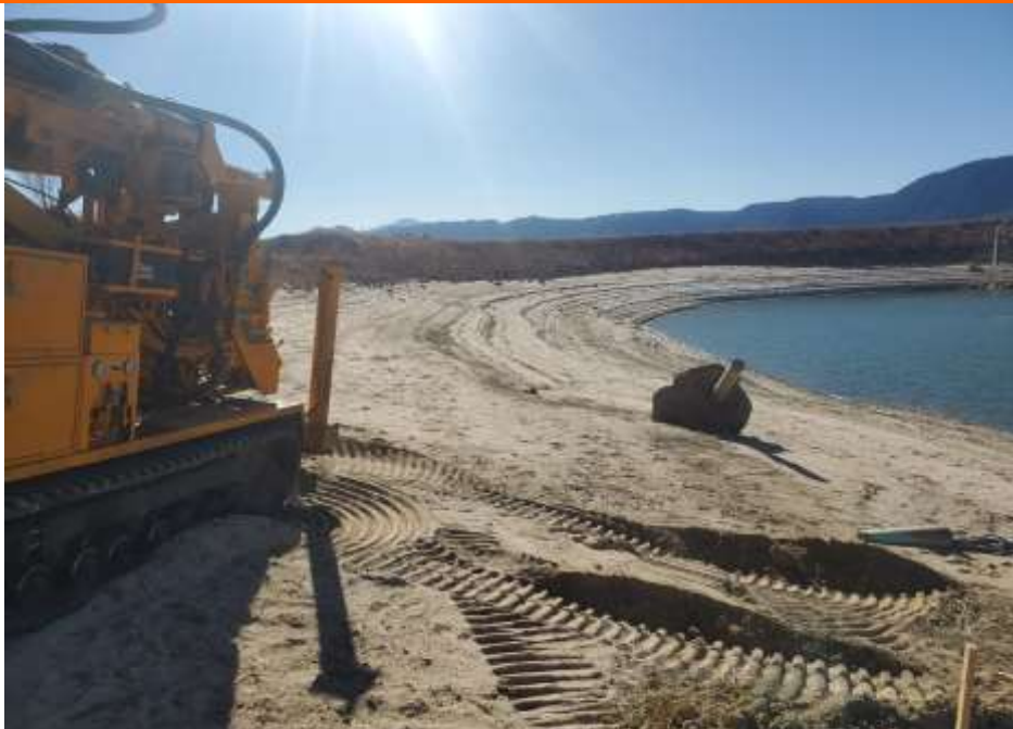
Near Boring SB-1 Facing Southwest
