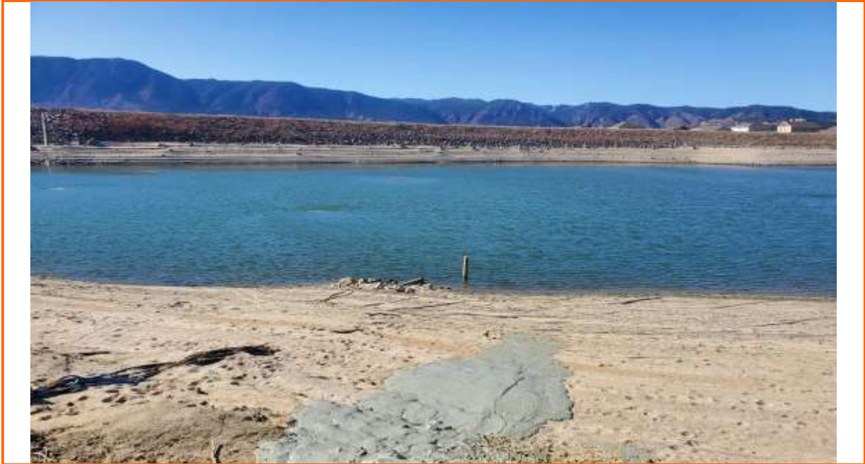
Near Boring SB-1 Facing Northwest
