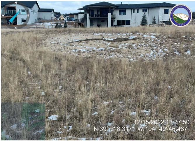
Photo 7: Address west-facing bare area along Detention Basin C embankment and remove temporary straw wattle.
