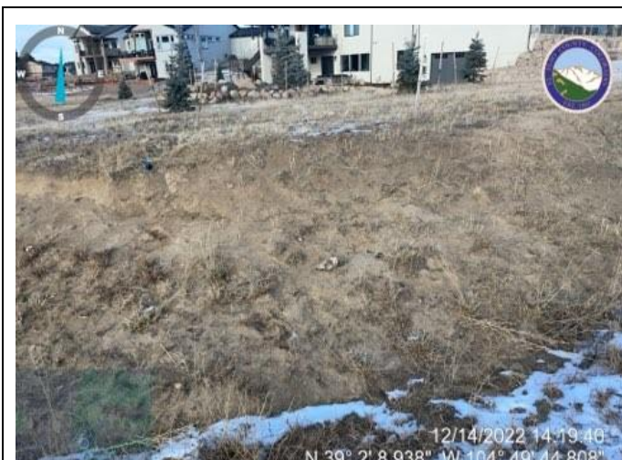
Photo 1: Stabilize slope of Swale K.
