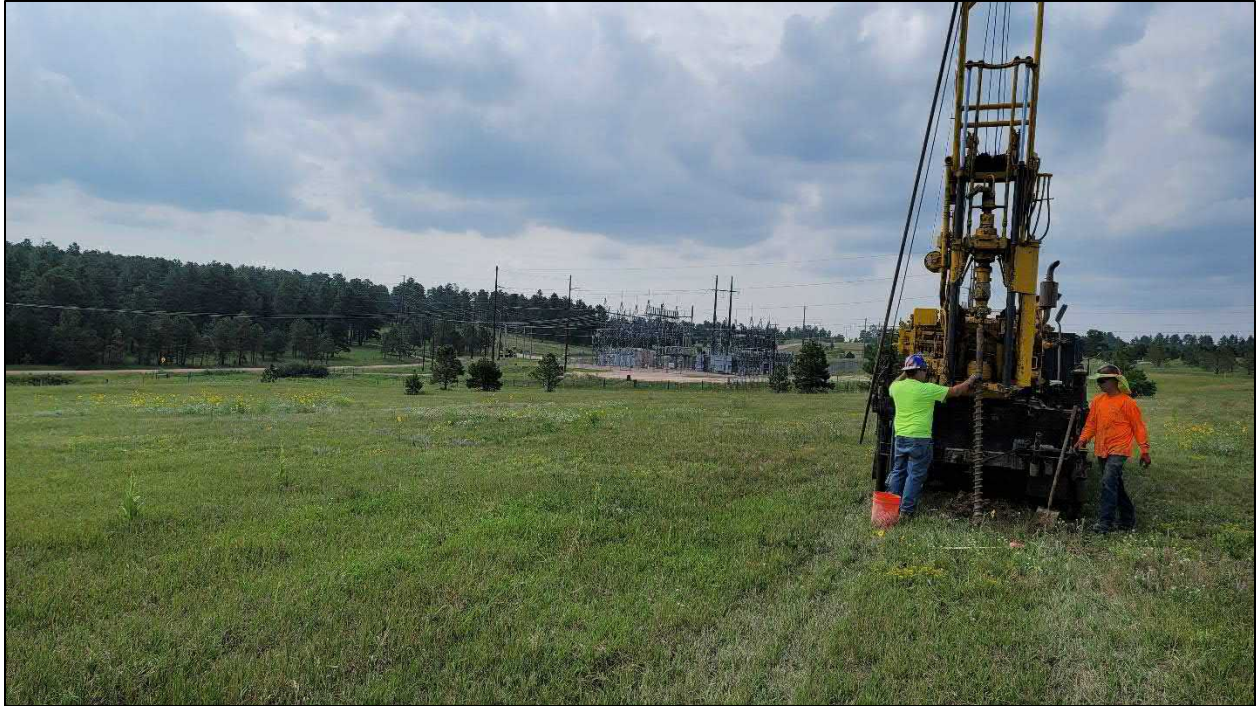
Photograph 2. Looking southeast from Boring B-13
