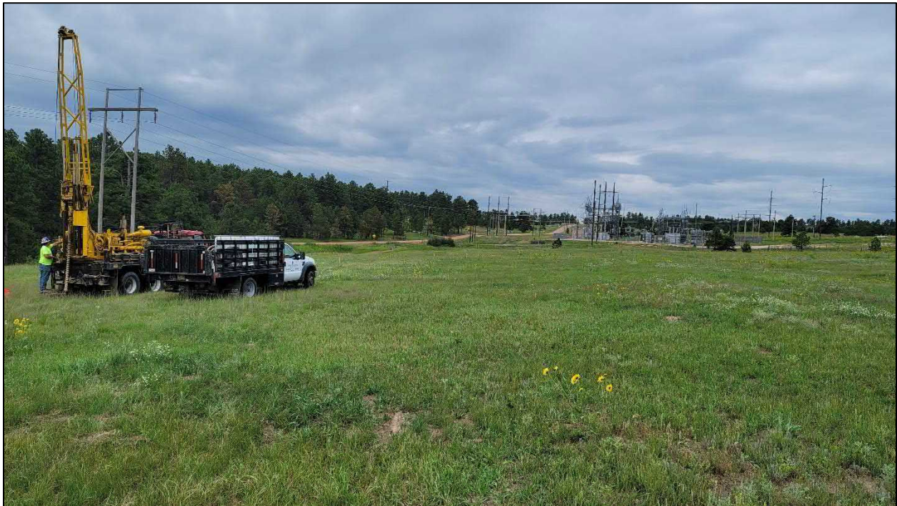
Photograph 1. Looking northeast from the southwest corner of proposed substation
