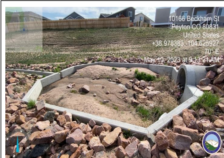
Photo 1: Clean out sediment and debris from Forebay.
