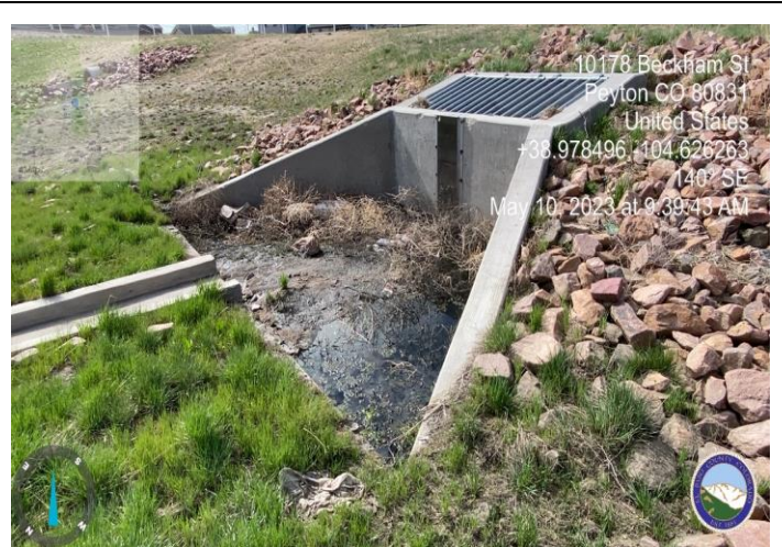
Photo 2: Clean out sediment and debris from outlet structure.
