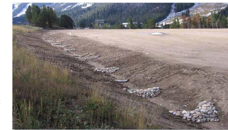
Photograph CD-1. Rock check dams in a roadside ditch. Photo courtesy of W.W.E.
