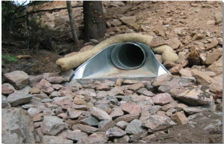
Photograph TOP-1. Riprap outlet protection.
