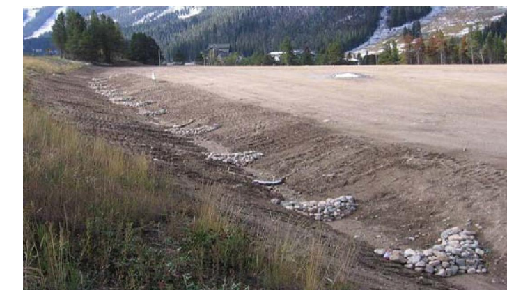
Photograph CD-1. Rock check dams in a roadside ditch. Photo courtesy of WWF.
