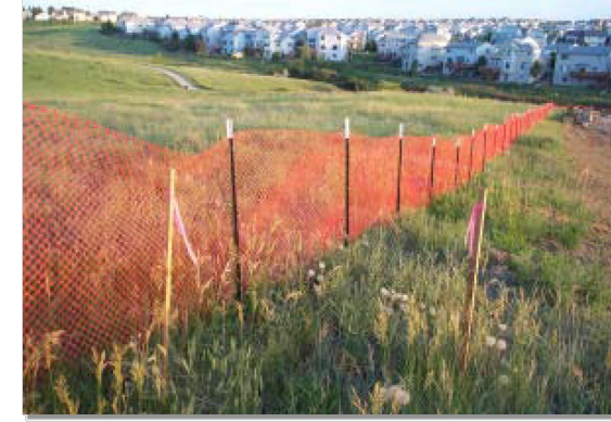
Photograph CF-1. A construction fence helps delineate areas where existing vegetation is being protected. Photo courtesy of Douglas County.
