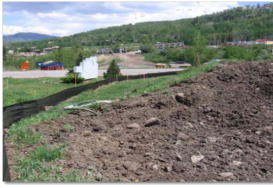
Photograph SP-1. A topsoil stockpile that has been partially revegetated and is protected by silt fence perimeter control.
