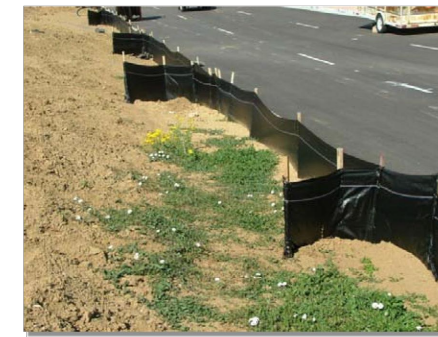
Photograph SF-2. When silt fence is not installed along the contour, a "J-hook" installation may be appropriate to ensure that the BMP does not create concentrated flow parallel to the silt fence. Photo courtesy of Tom Goe.
