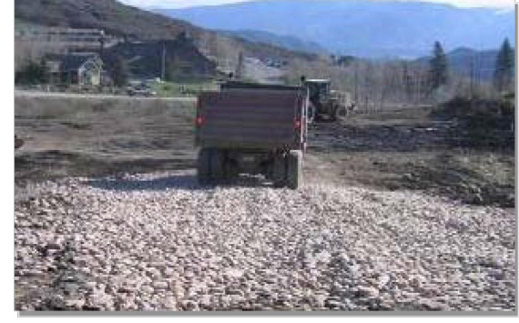
Photograph VTC-1. A vehicle tracking control pad constructed with properly sized rock reduces off-site sediment tracking.
