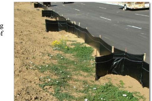
Photograph SF-2. When silt fence is not installed along the contour, a "J-hook" installation may be appropriate to ensure that the BMP does not create concentrated flow parallel to the silt fence. Photo courtesy of Tom Goe.
