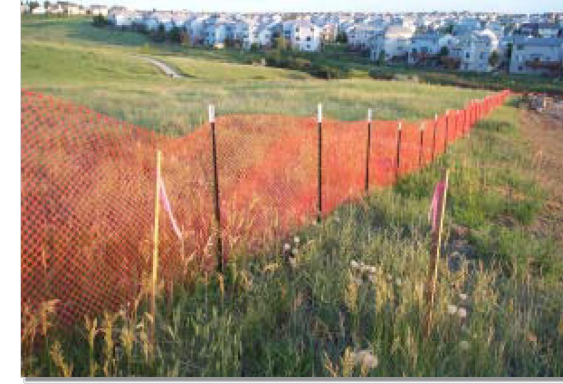
Photograph CF-1. A construction fence helps delineate areas where existing vegetation is being protected. Photo courtesy of Douglas County.
