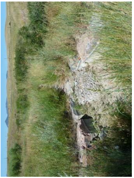
CONSTRUCTED ROCK CROSS VANE
