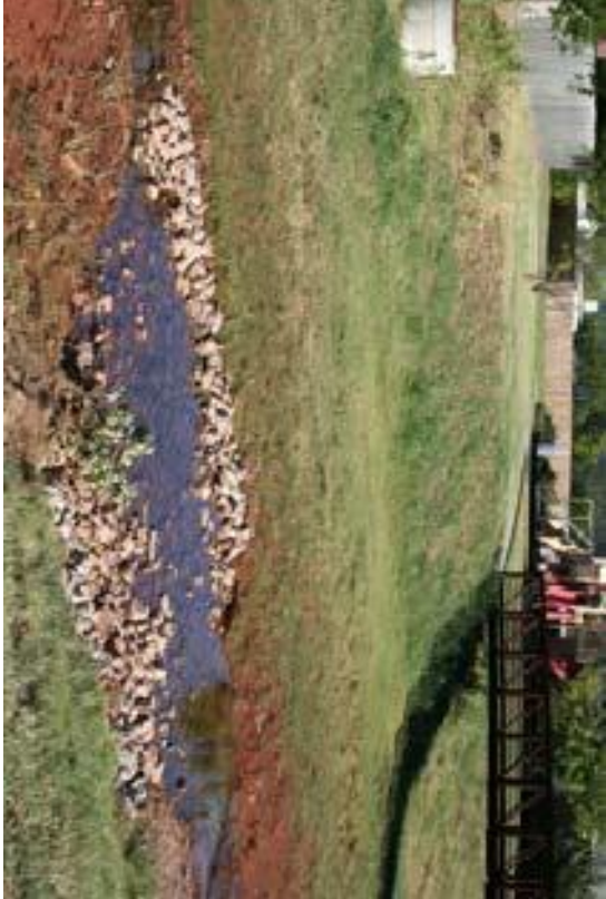
CONSTRUCTED RIFFLE DROP STRUCTURE
