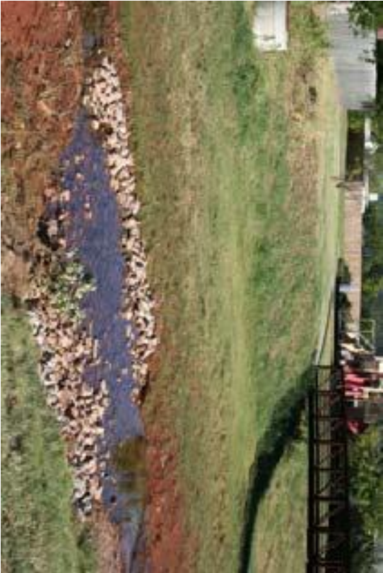
CONSTRUCTED RIFFLE DROP STRUCTURE
