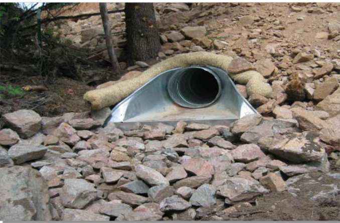
Photograph TOP-1. Riprap outlet protection.
