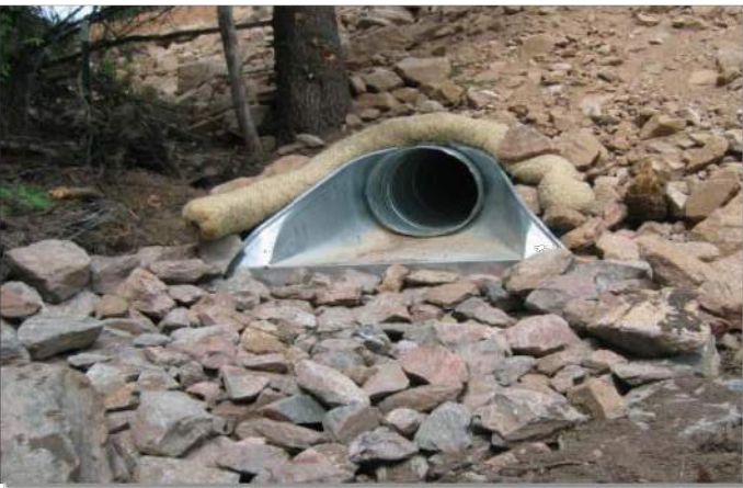
Photograph TOP-1. Riprap outlet protection.
