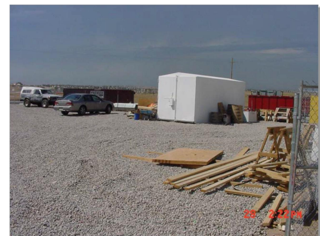
Photograph SSA-1. Example of a staging area with a gravel surface to prevent mud tracking and reduce runoff. Photo courtesy of Douglas County.
