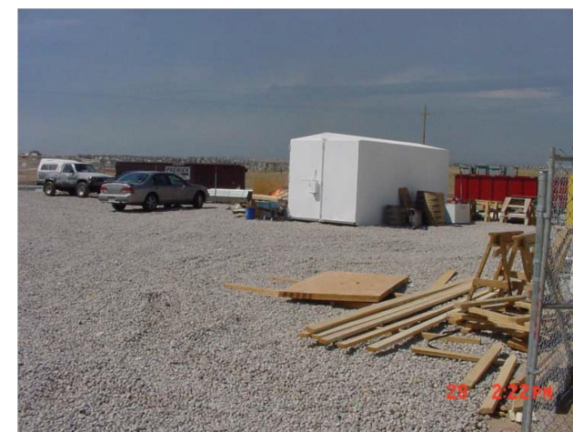
Photograph SSA-1. Example of a staging area with a gravel surface to prevent mud tracking and reduce runoff. Photo courtesy of Douglas County.
