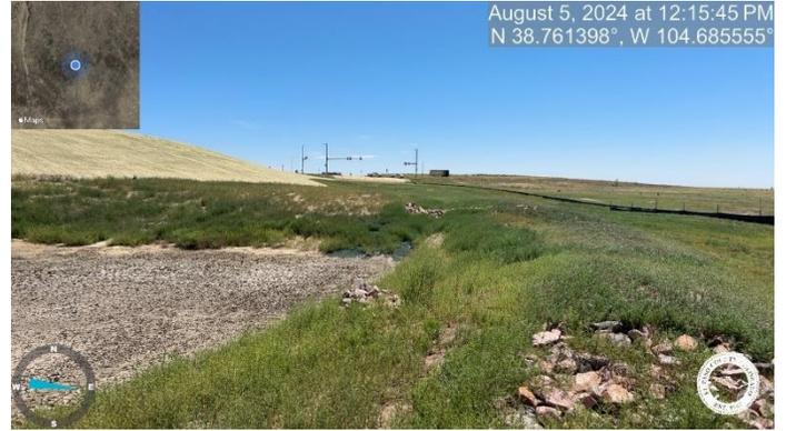
**Photo 2:** Rock checks have been added to pond. Reflect the change on the Addendum to the Drainage Letter.
