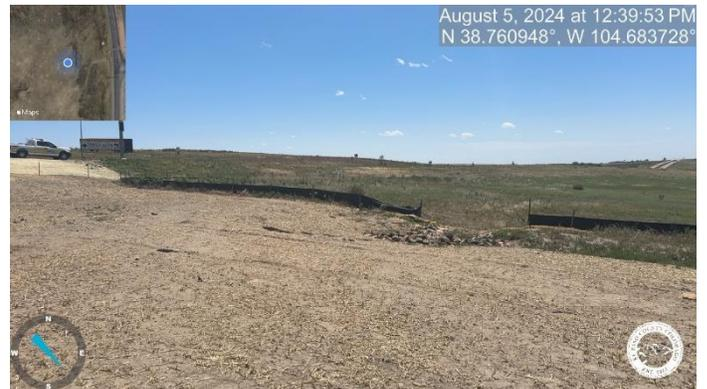
**Photo 4:** Rock checks have been installed near site entrance. Reflect the change on the Addendum to the Drainage Letter.
