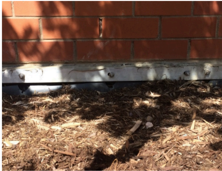
Photograph B-2. The impermeable membrane in this photo has ripped from the bolts due to placement of the media without enough slack in the membrane.
