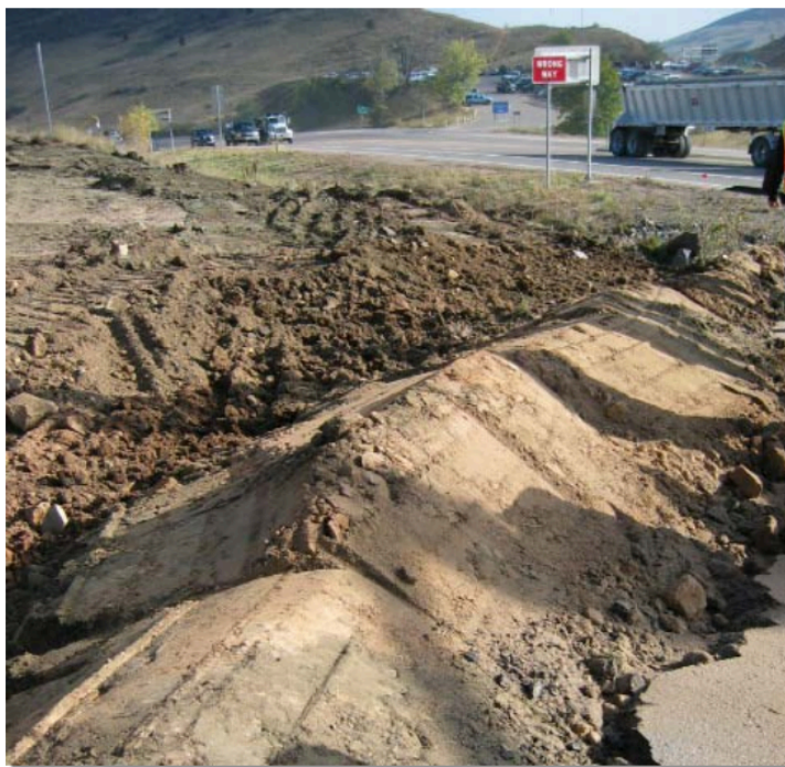
Photograph ED/DS-1. Example of an earth dike used to divert flows at a construction site. Photo courtesy of CDOT.
