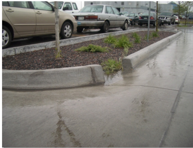
Photograph B-4. The curb cut shown allows flows to enter this rain garden while excess flows bypass the facility.
