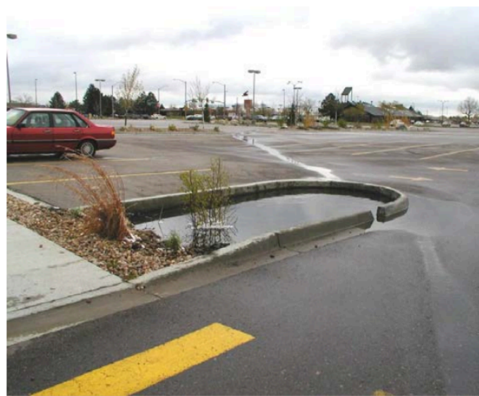
Photograph B-4. Runoff passed the upgradient rain garden, shown Photo B-3, and flooded this downstream rain garden.
