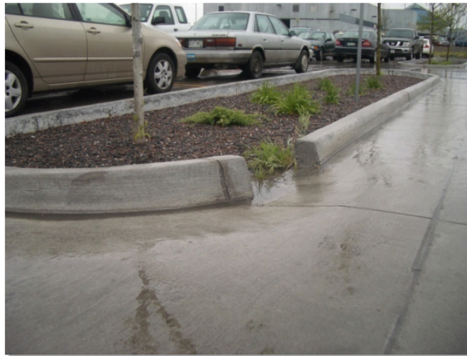
Photograph B-4. The curb cut shown allows flows to enter this rain garden while excess flows bypass the facility.
