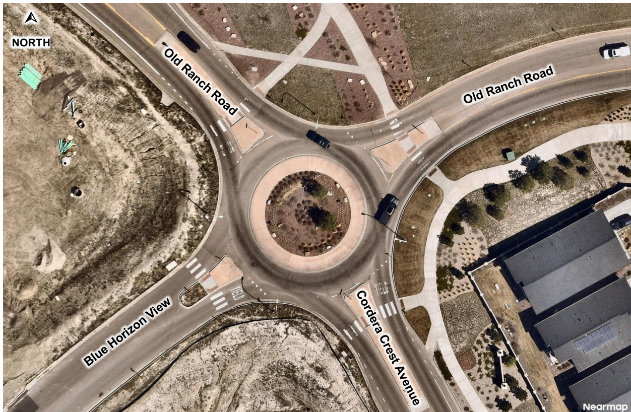
Blue Horizon View/Old Ranch Road and Old Ranch Road/Cordera Crest Avenue (#1)
