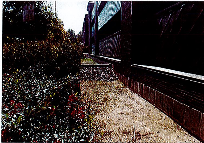
Photograph SF-1. This sand filter, constructed on two sides of a parking garage, is accessible for maintenance, yet screened from public view by a landscape buffer.
