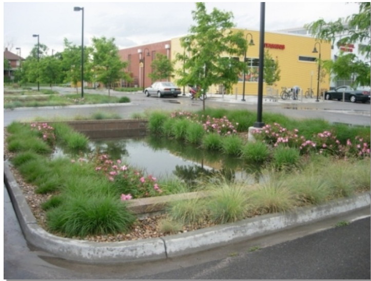
Photograph EDB-4. A series of landscape islands connected by culverts provide water quality and flood control for this site.
