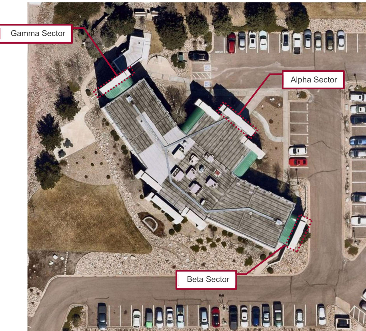
Figure 2a Overall Building
