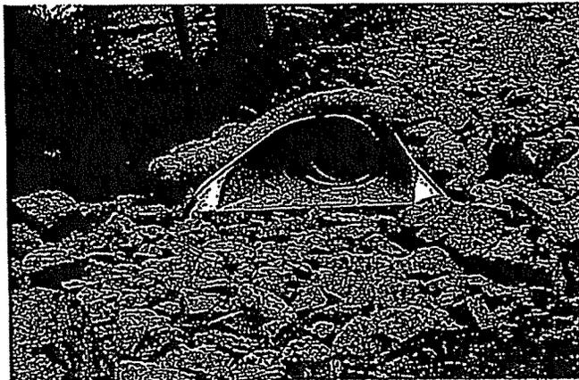
Photograph TOP-1. Riprap outlet protection.
