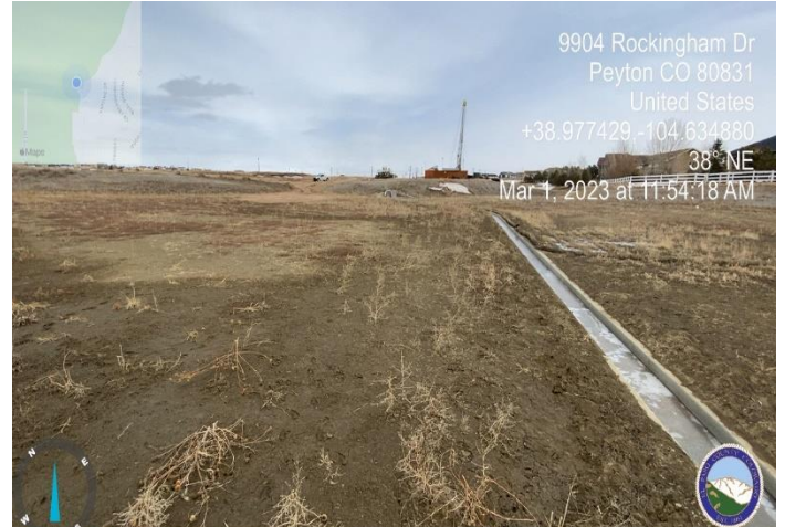
Photo 2: Regrade pond bottom to top of trickle channel curb with a 3% slope towards trickle channel for positive drainage. Stabilize pond bottom where disturbance occurred.
