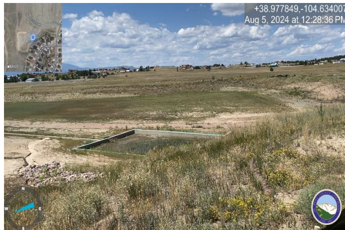
Photo 3: Remove sediment, vegetation, and debris from forebay.
