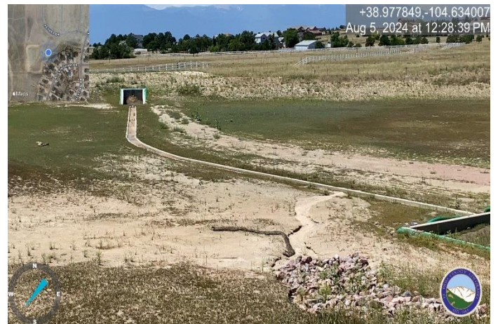
Photo 4: Remove sediment, vegetation, and debris from trickle channel and outlet structure.
