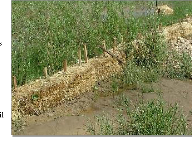
Photograph SBB-1. Straw bale barrier used for perimeter control. Photo courtesy of Tom Gore.
