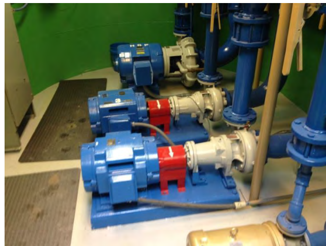
Figure 6: PBHMD Booster Pumps
