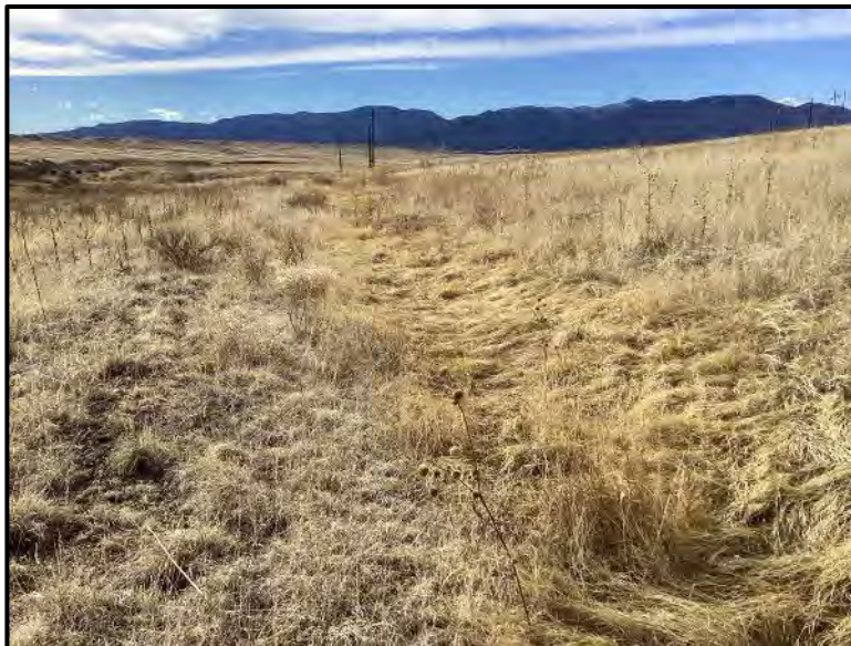
Photo 2. A west-facing view of a constructed upland drainage swale located within the Project Area.
