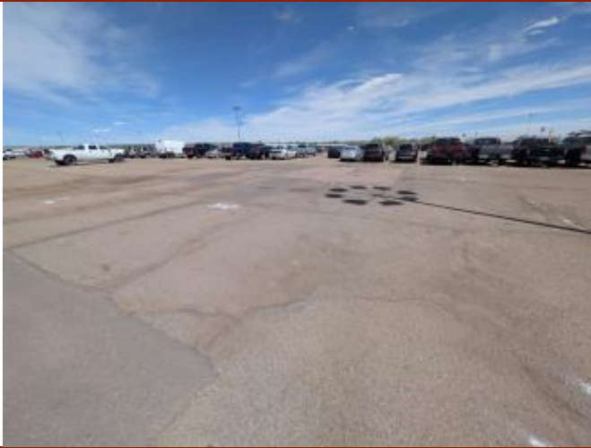
Photo 5 – North Building Area Direction: Northeast
