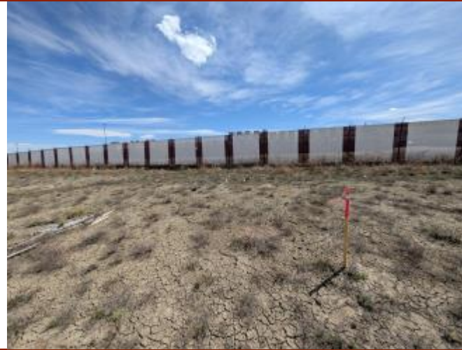
Photo 14 – South Building Area Direction: South
