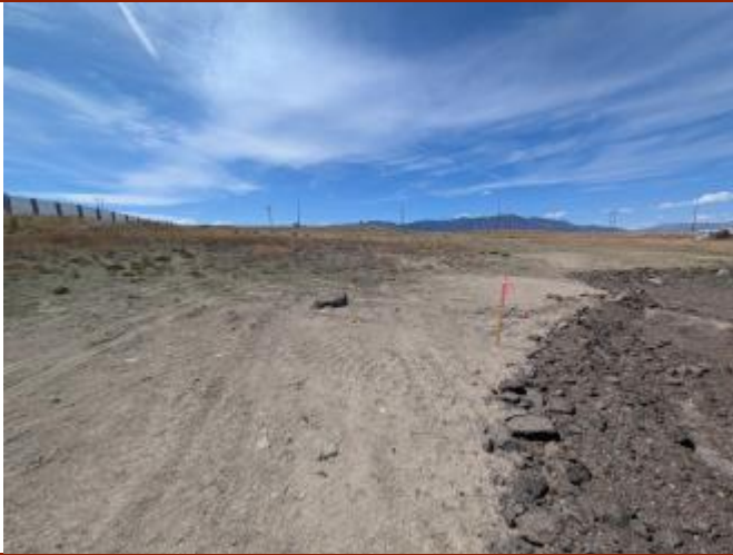
Photo 13 – South Building Area Direction: Northwest
