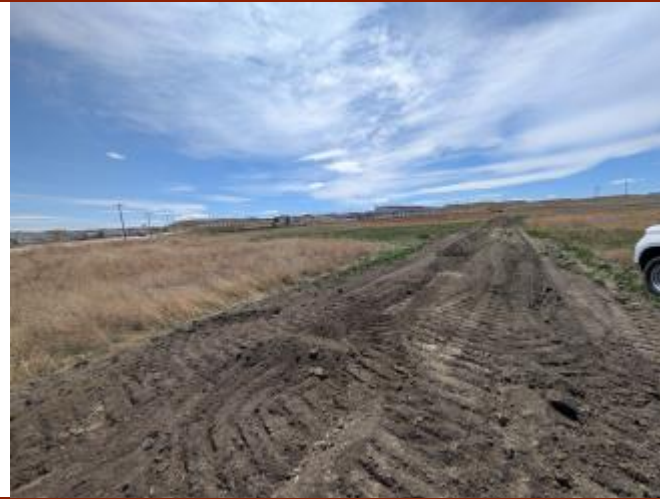
Photo 6 – South Building Area Direction: Southwest
