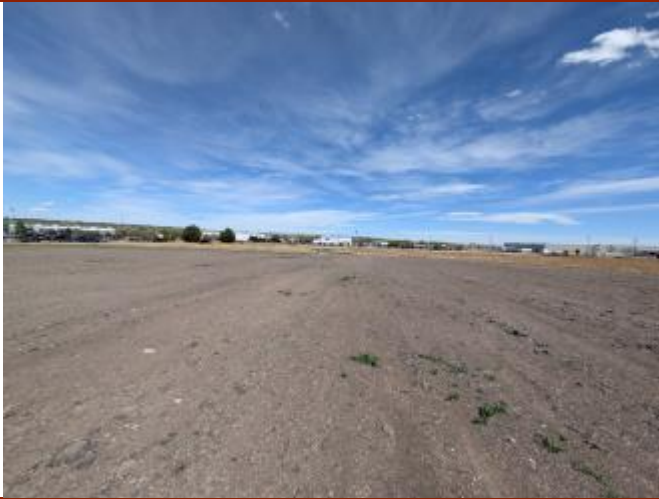
Photo 17 – South Building Area Direction: East
