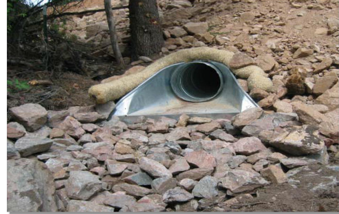
Photograph TOP-1. Riprap outlet protection.
