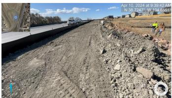
Photo 9: Install Type M soil riprap with 3"-4" topsoil revegetated with seed mix. Current riprap does not consist of all Type M aggregate. Reference Sheet 28 of the Construction Drawings.
