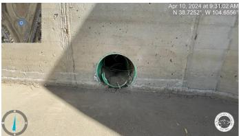
Photo 25: Forebay H: Energy Dissipator Baffle was installed at 6'5" from the inflow pipe. Plans call for a distance of 7'6". Change structure to match approved plans or justify change in the As-builts/Drainage Report. Reference Sheet 28 of the Construction Drawings.
