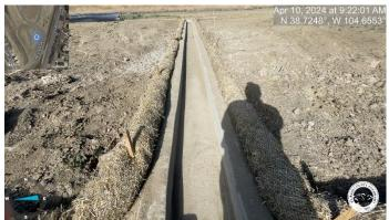
Photo 19: Forebay J: Forebay measures 13'x17'2". Plans call for 23'x19'. Change structure to match approved plans or justify change in the As-builts/Drainage Report. Reference Sheet 28 of the Construction Drawings.
