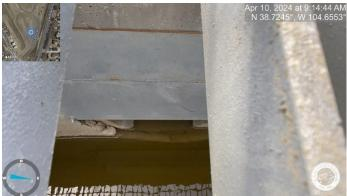
Photo 13: Pond Outlet Structure: Install orifice plate with the proper sized holes. Reference Sheet 30 of the Construction Drawings.
