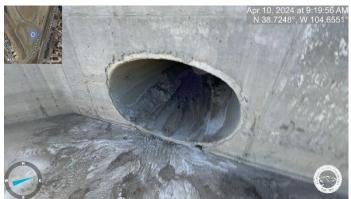
Photo 15: Forebay J: Energy Dissipator Baffle was installed at 5'4" from the inflow pipe. Plans call for a distance of 7'6". Change structure to match approved plans or justify change in the As-builts/Drainage Report. Reference Sheet 28 of the Construction Drawings.
