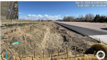
Photo 5: Box Culvert: Install riprap pad at culvert inflow point. Reference Sheet 29 of the Construction Drawings.
