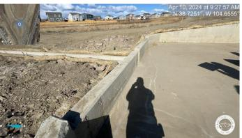
Photo 23: Forebay H: Forebay H: Install 16'x2'6" trickle channel at front of forebay per the approved plans. Reference Sheet 28 of the Construction Drawings.
