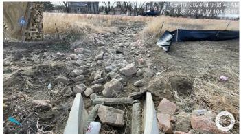
Photo 11: Pond Outfall: Confirm outfall elevation allows for positive drainage.
