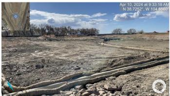
Photo 27: Forebay J: Forebay measures 18'5"x26'10". Plans call for 23'x19'. Change structure to match approved plans or justify change in the Asbuilts/Drainage Report. Reference Sheet 28 of the Construction Drawings.
