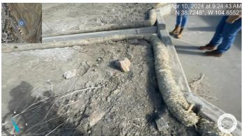
Photo 17: Forebay J: Slot opening measures 10.5". Plans call for 7.8". Change structure to match approved plans or justify change in the As-builts/Drainage Report. Reference Sheet 28 of the Construction Drawings.
