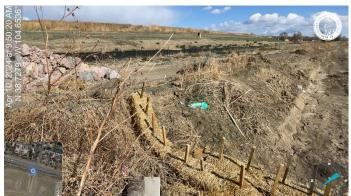
Photo 3: Inlets that need to be cleaned of sediment and debris are marked with green paint.
