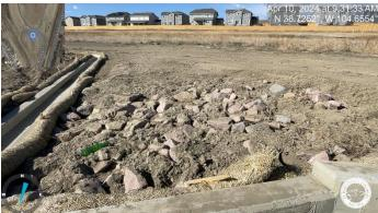
Photo 21: Forebay H: Fill in soil riprap to be free of voids and flush with grade.
