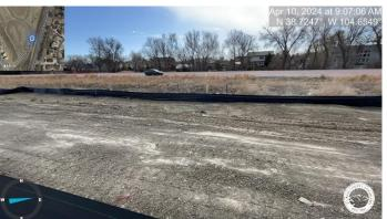
Photo 7: Box Culvert: Fine grade culvert outfall to allow for positive drainage and stabilize.
