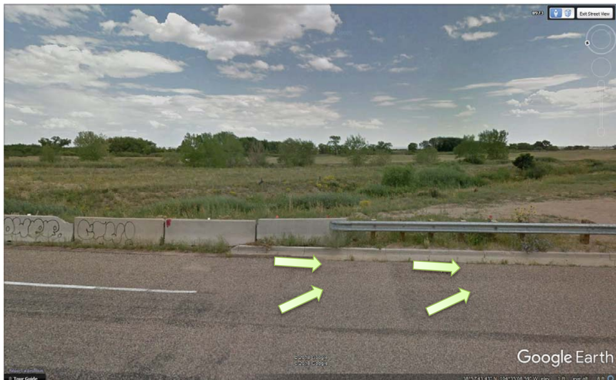
Google Streetview at the upstream end of the gutter line (south side of Bennett Ranch drainageway crossing). Transition from block to 6 inch curb.
