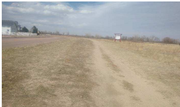
Figure A3. Project area looking north along Eastonville Road right-of-way.
