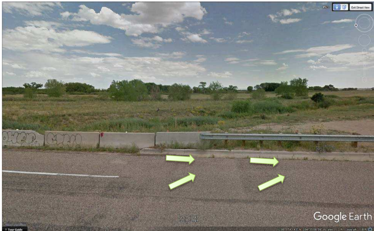
Google Streetview at the upstream end of the gutter line (south side of Bennett Ranch drainageway crossing). Transition from block to 6 inch curb.
