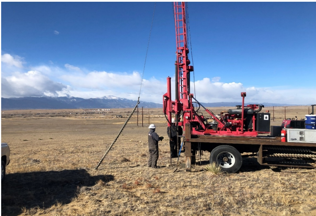
DRILLING BORING B-9 - LOOKING NORTHWEST
