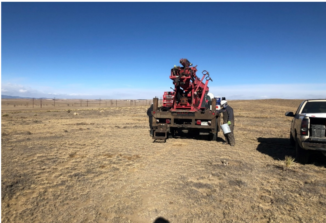
DRILLING BORING B-11 - LOOKING NORTH
