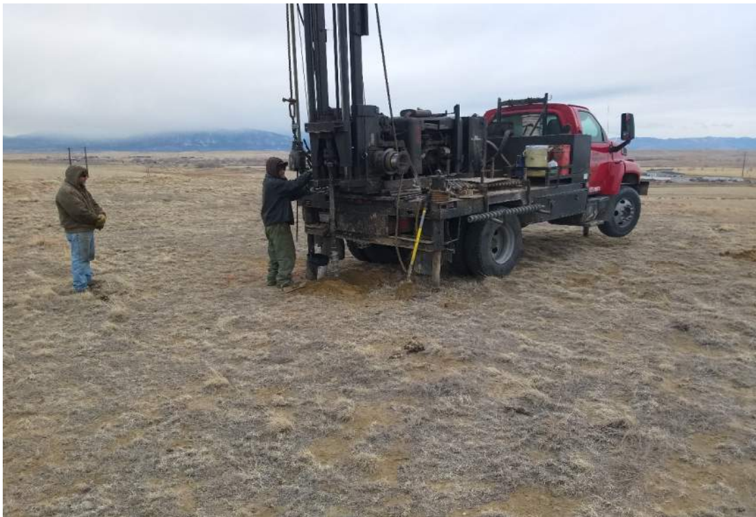
DRILLING BORING B-4 - LOOKING WEST
