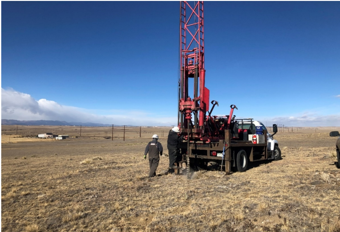
DRILLING BORING B-10 - LOOKING NORTHWEST
