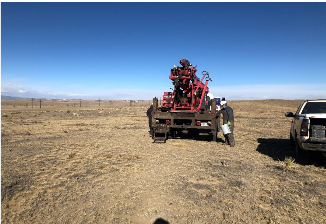
DRILLING BORING B-11 - LOOKING NORTH
