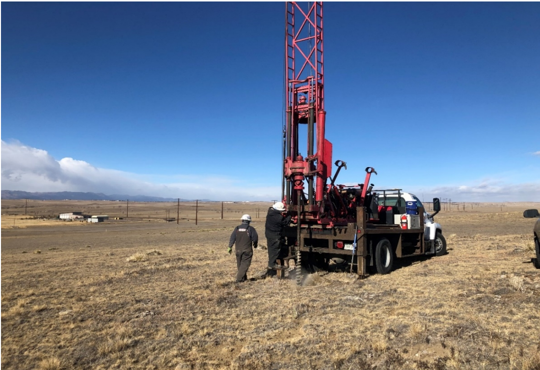
DRILLING BORING B-10 - LOOKING NORTHWEST
