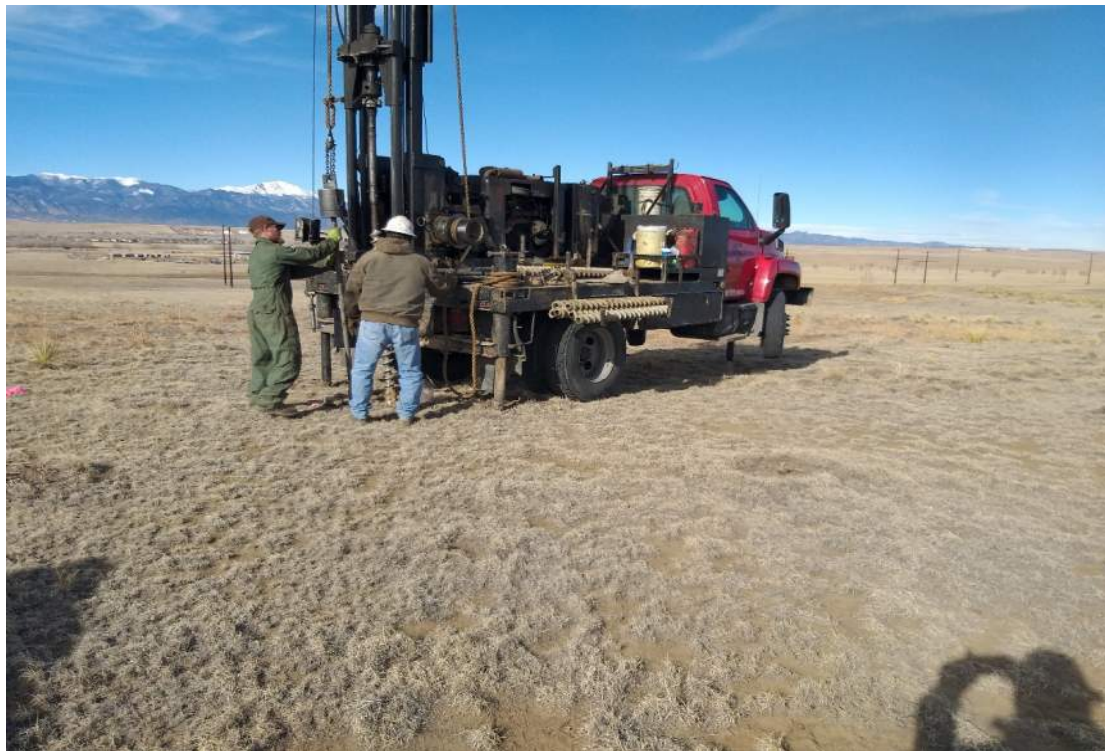
DRILLING BORING B-6- LOOKING NORTHWEST
