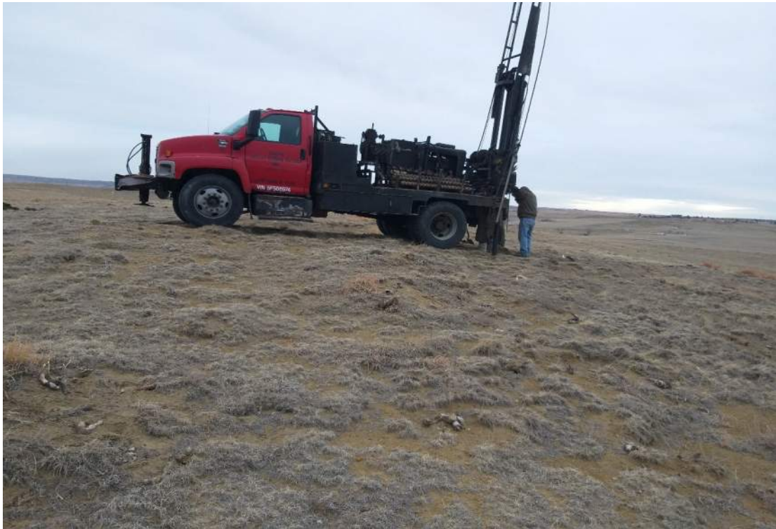
DRILLING BORING B-5 - LOOKING NORTH
