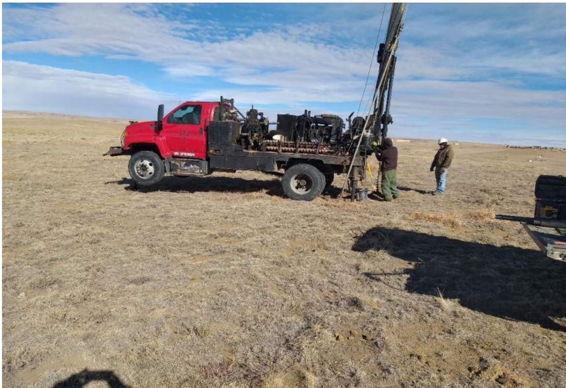
DRILLING BORING B-2 - LOOKING NORTHEAST
