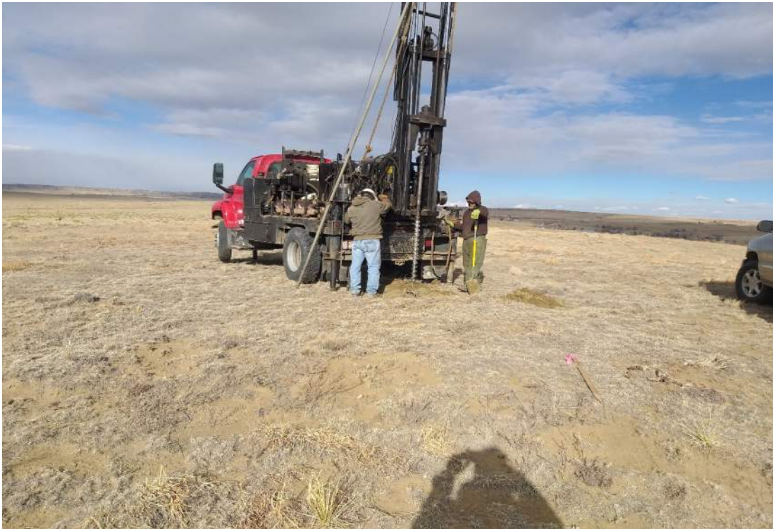
DRILLING BORING B-3 - LOOKING NORTH
