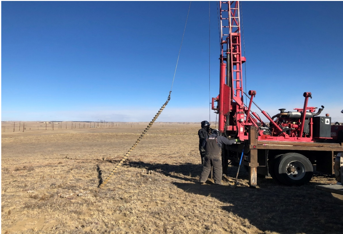
DRILLING BORING B-8 - LOOKING NORTH
