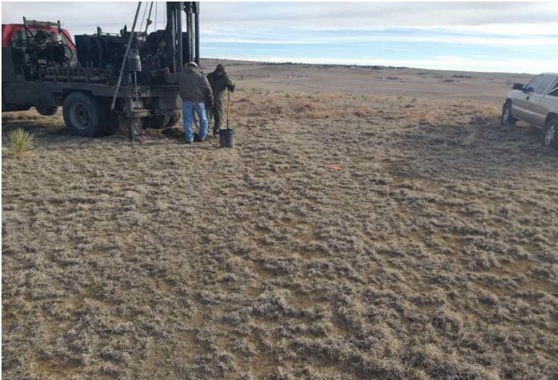
DRILLING BORING B-7 - LOOKING NORTHEAST
