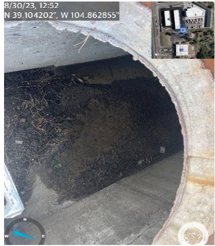
Photo 6: Clean out southeast inlet at STA 3+30.09.
