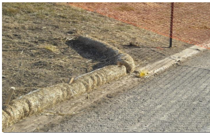
Photographs SCL-1 and SCL-2. Sediment control logs used as 1) a perimeter control around a soil stockpile; and, 2) as a "J-hook" perimeter control at the corner of a construction site.
