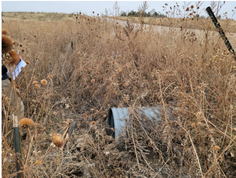
Figure 7: Culvert Entrance, 30" diameter.
