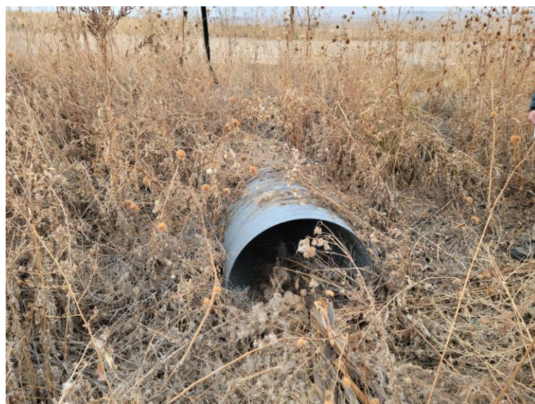
Figure 8: Culvert Exit, 30" diameter.
