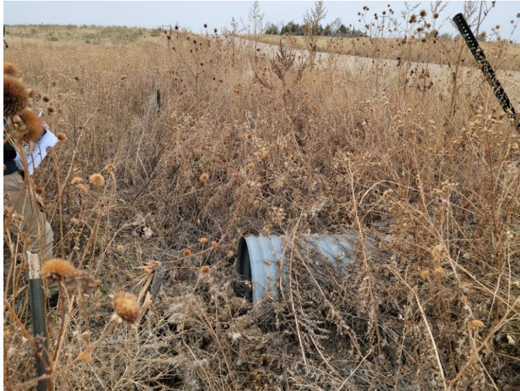
Figure 7: Culvert Entrance, 30" diameter.
