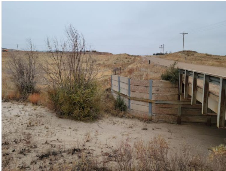
Figure 9: Creek Entrance under S. Franceville Coal Mine Rd, site shown in the distance to the South. Drainage path shown along roadside draining into the creek.
