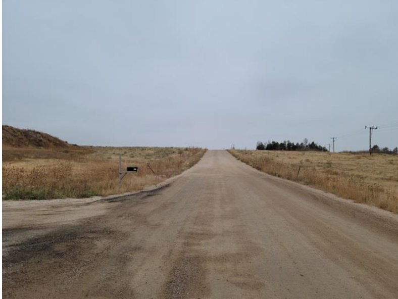
Figure 1: S. Franceville Coal Mine Rd. in front of site access driveway facing South.
