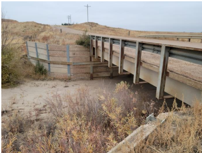
Figure 10: Creek Entrance under S. Franceville Coal Mine Rd.
