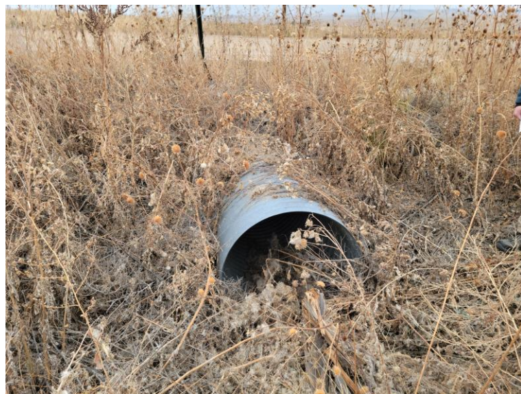
Figure 8: Culvert Exit, 30" diameter.
