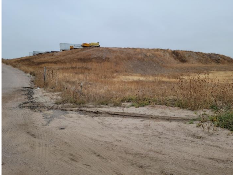
Figure 3: S. Franceville Coal Mine Rd. in front of site access driveway facing East toward the site.
