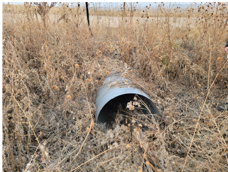
Figure 8: Culvert Exit, 30" diameter.
