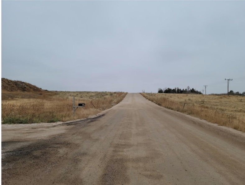
Figure 1: S. Franceville Coal Mine Rd. in front of site access driveway facing South.
