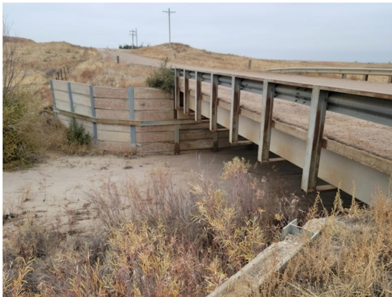
Figure 10: Creek Entrance under S. Franceville Coal Mine Rd.
