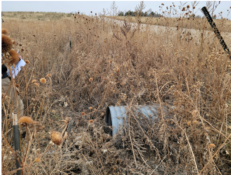
Figure 7: Culvert Entrance, 30" diameter.
