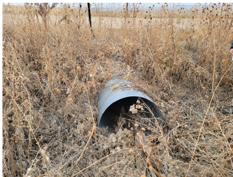
Figure 8: Culvert Exit, 30" diameter.
