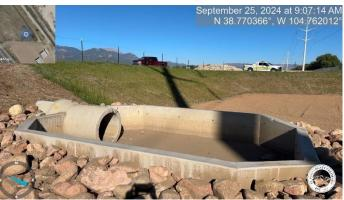
**Photo 1:** Install ditch or reflect change on as builts.
